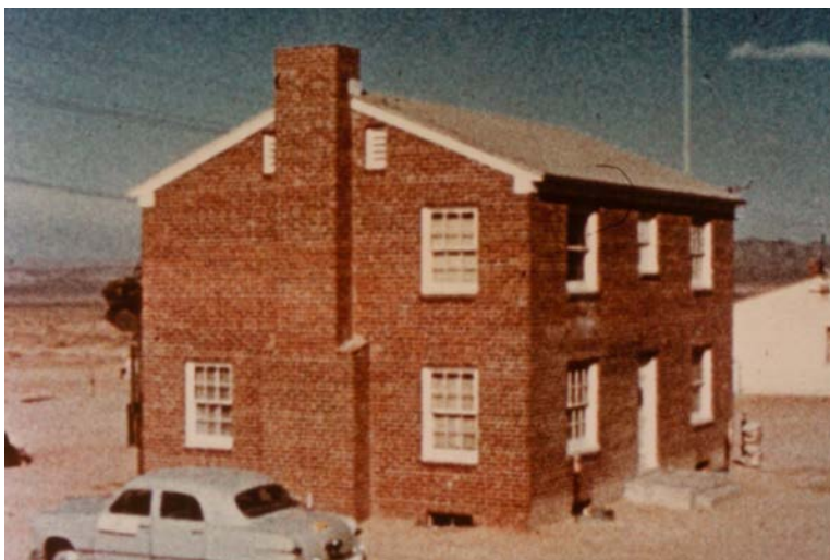
Operation Teapot contained another test, called Apple II, conducted on May 5, 1955, that had an associated civil defense program called Operation Cue. A brick two-story house and a wooden two-story house, along with three bungalows (all built with different construction materials) were part of a small town that featured other municipal elements, including a radio broadcast, propane, and electrical transfer stations. Photo courtesy the National Archives and Records Administration.
