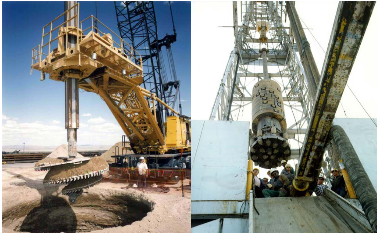
Large emplacement hole and large-diameter drill bits circa 1990. Photo courtesy the National Nuclear Security Administration/Nevada Site Office.
